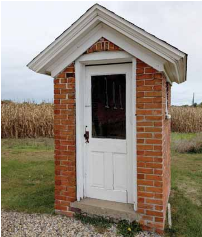
A two-seater outhouse at Spring Creek School. Photo by Bryan Lawler
