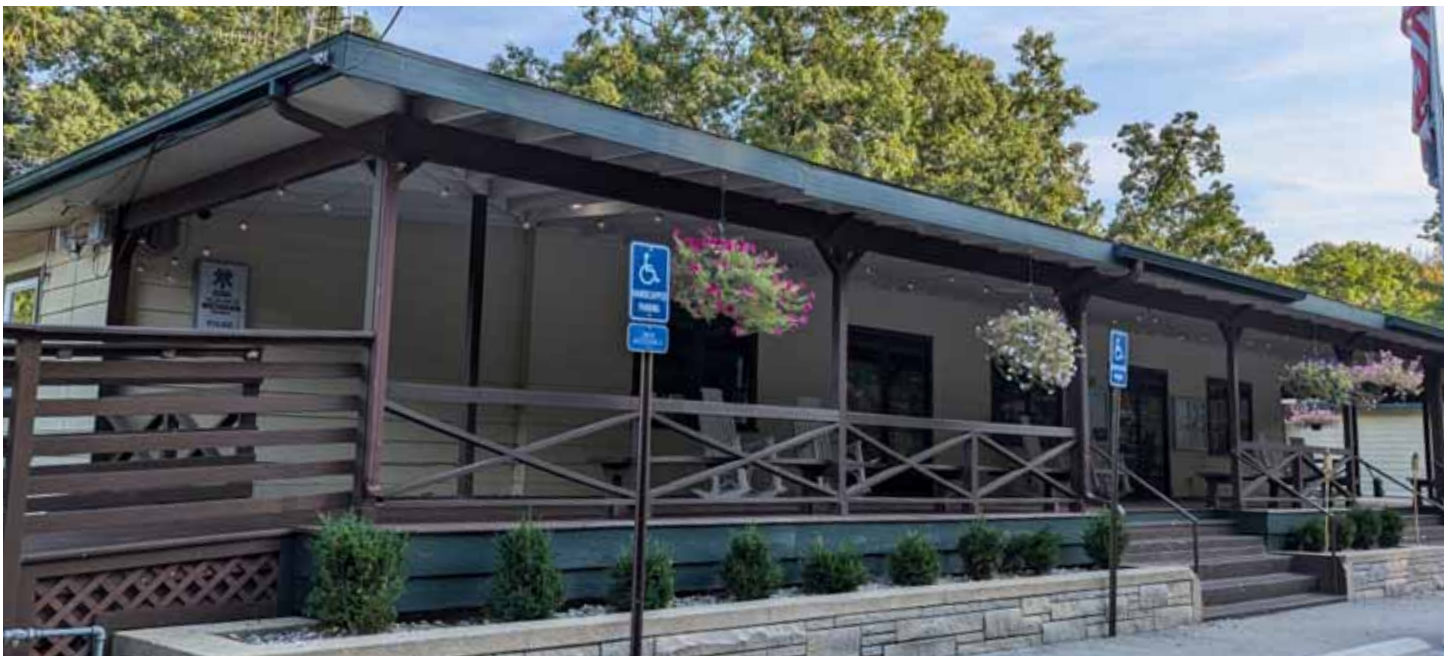
The Michiana Village Hall, built in 1947, is undergoing restoration. Photo by Bryan Lawler.
