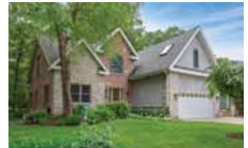
19660 DOGWOOD DR, NEW BUFFALO Custom-built home says quality. Real stone and brick 4 br, 2.5 ba 2-story. $900,000 CHRISTINA KELLY 269.469.8300
